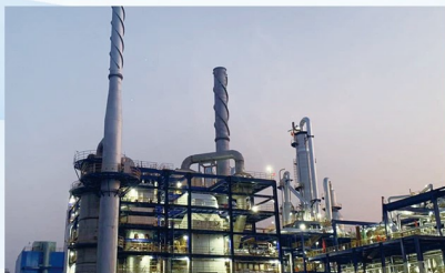
waste liquid ( heavy ends) | 32t/h
